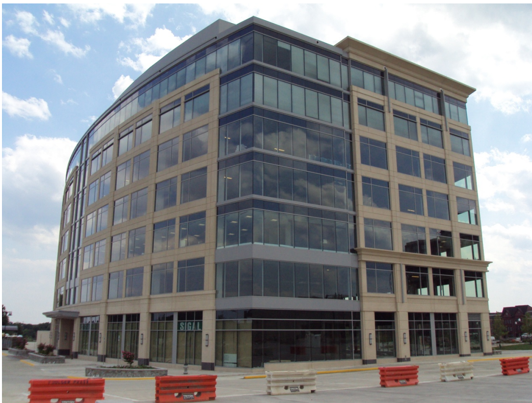
Figure 6: View of South-West Corner
